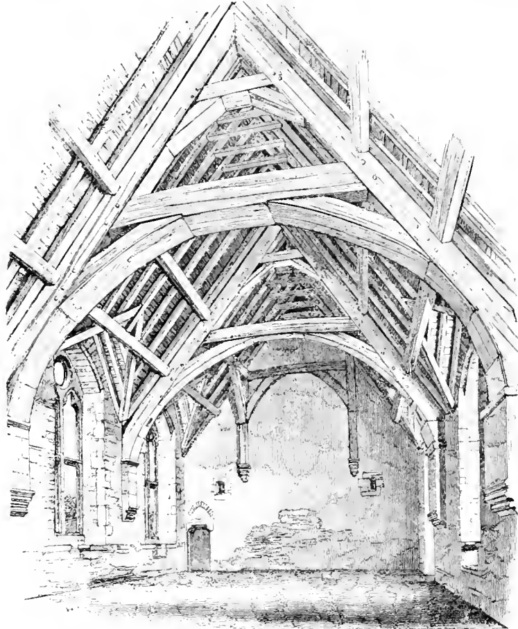
ROOF: WITH COLLAR BEAMS AND BRACES (KNEE RAFTERS), 13TH CENTURY; HALL OF STORESAY CASTLE, SHROPSHIRE.
